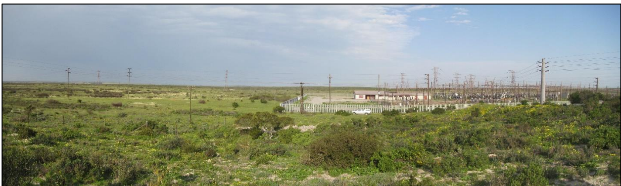
Figure 4: View towards the east of the Blouwater Substation and, to its left, the proposed Alternative A distribution substation site. Alternative B lies further east in the distance, while Alternative C is out of view towards the left.
