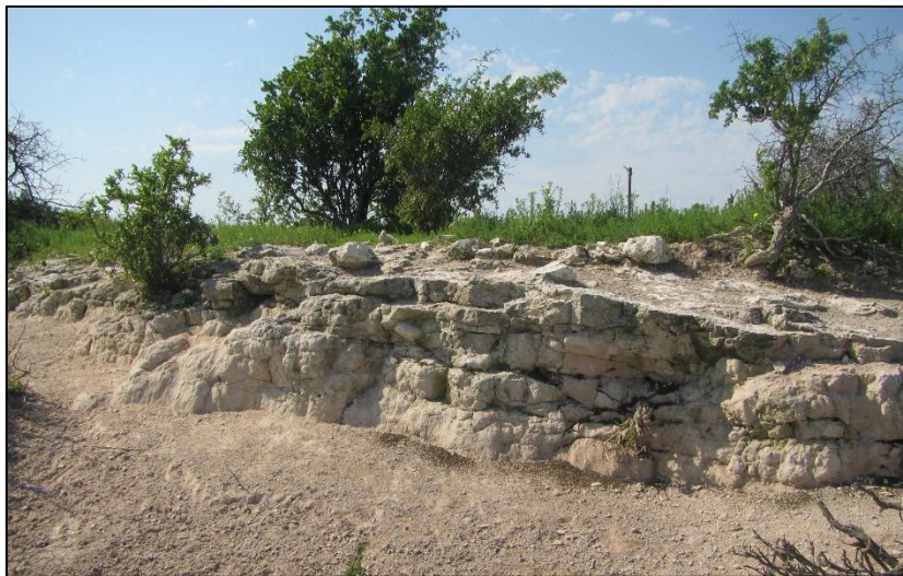
Figure 28: Cutting through calcrete along the east side of the R27 within corridor occupied by all three transmission alternatives.
