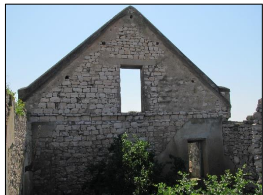
Figure 26: Inside view of the still standing north gable showing the concrete lintel above the loft door.
